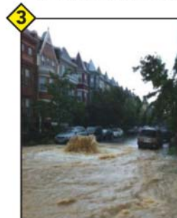
▲ Flooding at 1st and V Streets NW
