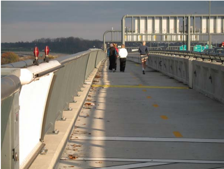
Figure 2: Woodrow Wilson Bridge Trail
