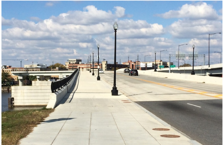
Figure 10: 11 th Street Bridge
