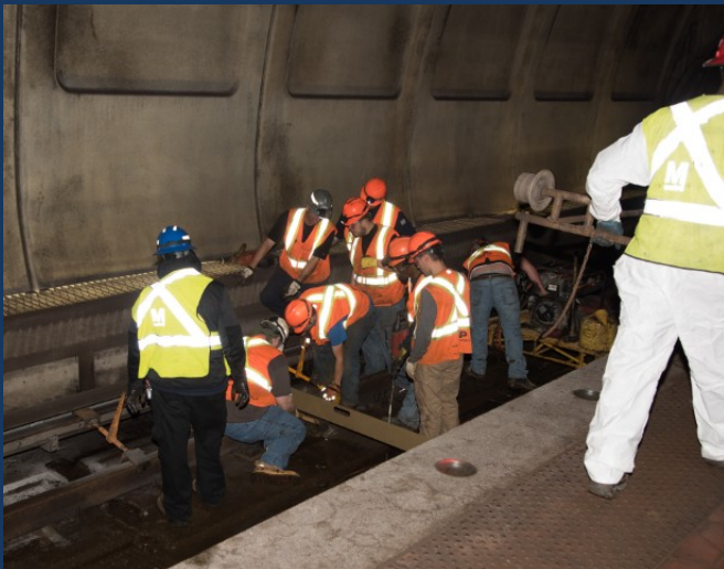
Photo of Trackwork at the Bethesda Station
