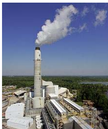
The largest fossil-fueled power station in Virginia, Dominion Virginia Power's Chesterfield facility, burns coal, oil and natural gas. (Photo courtesy Dominion Virginia Power)
