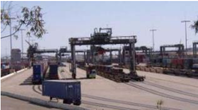
From Port to Rail
