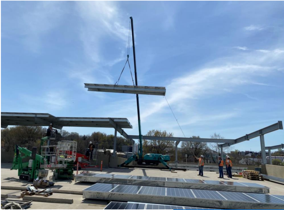
Crane lifts a row of panels at Anacostia Garage (April 2022)
