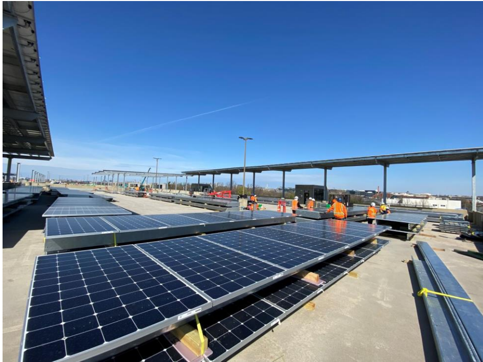
Solar Installation at Anacostia Garage (April 2022)
