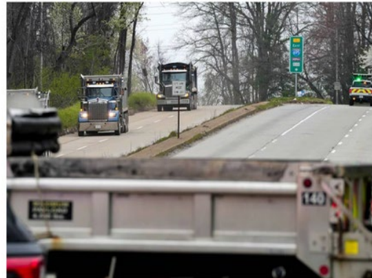
Trucks coming back from the way of the Francis Scott Key Bridge, which was toppled by a massive container ship on March 26, 2024. The loss of the bridge, a key segment in the Baltimore Beltway, has left drivers looking for other routes around the city or to and from the Port of Baltimore. (Kylie Cooper/The Baltimore Banner)
