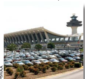
Dulles Corridor Rapid Transit
