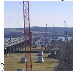
Woodrow Wilson Bridge
