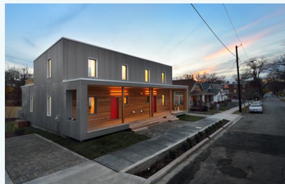
The Empowerhouse, designed and built by the New School and Stevens Institute of Technology team
