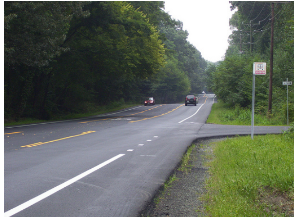
Figure 72: Lawyers Road After Road Diet/VDOT
