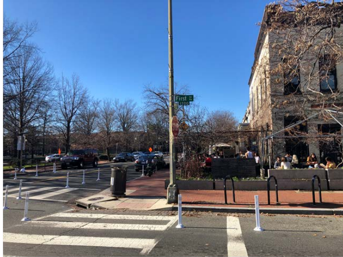
Figure 45: Flexpost Bulbouts/TPB/Michael Farrell
