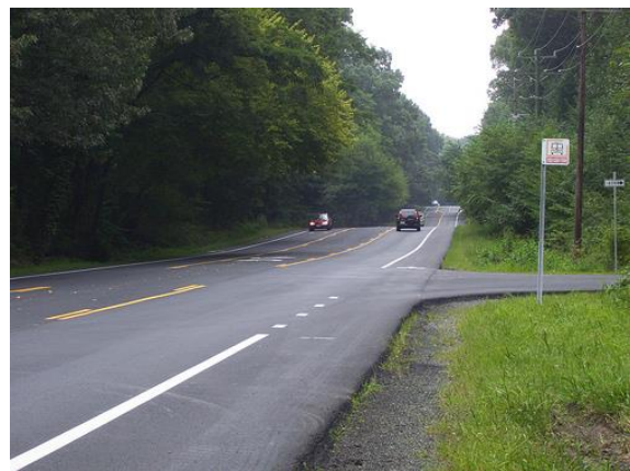
Figure 72: Lawyers Road After Road Diet/VDOT
