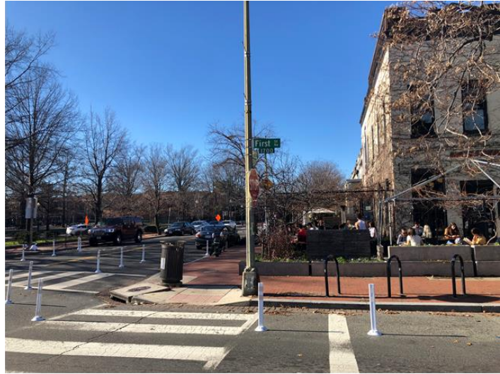
Figure 45: Flexpost Bulbouts/TPB/Michael Farrell
