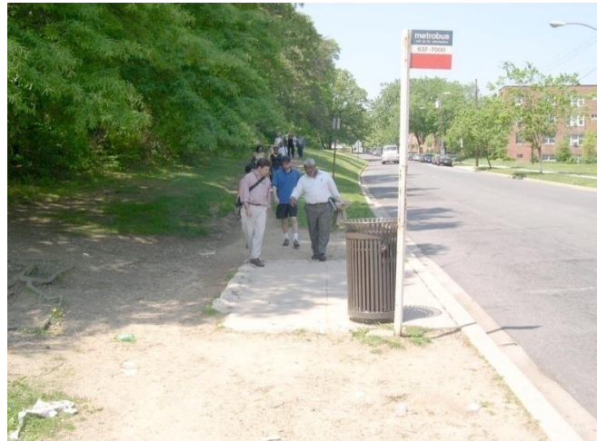
Figure 60: Missing Sidewalk/TPB/Michael Farrell
