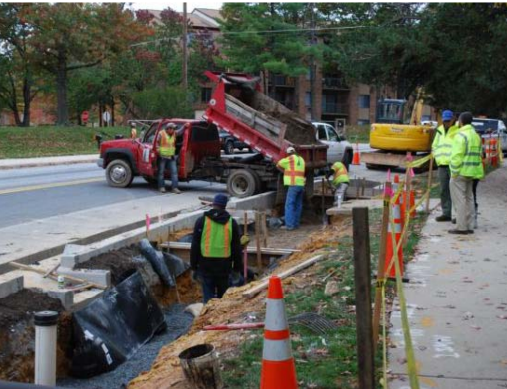
Montgomery County stormwater control 'bump out' under construction
