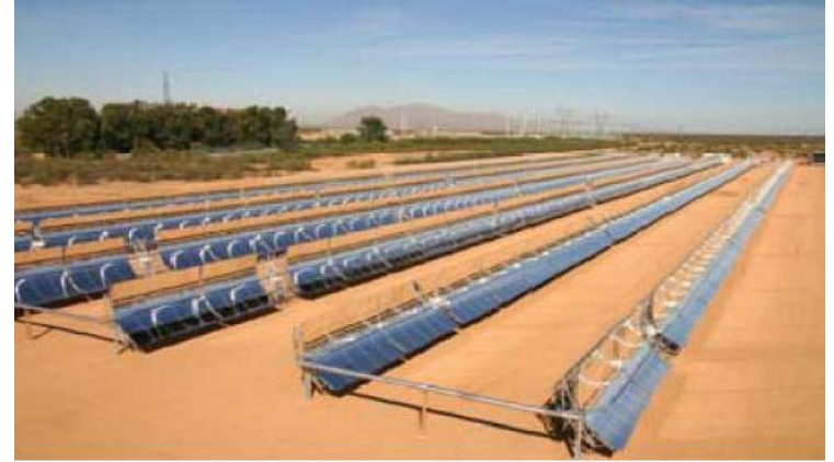
APS' Saguaro Power Plant, about 30 miles north of Tucson.
