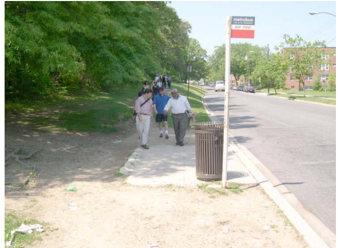
Figure 1: Missing sidewalk near Ft. Totten Metro
