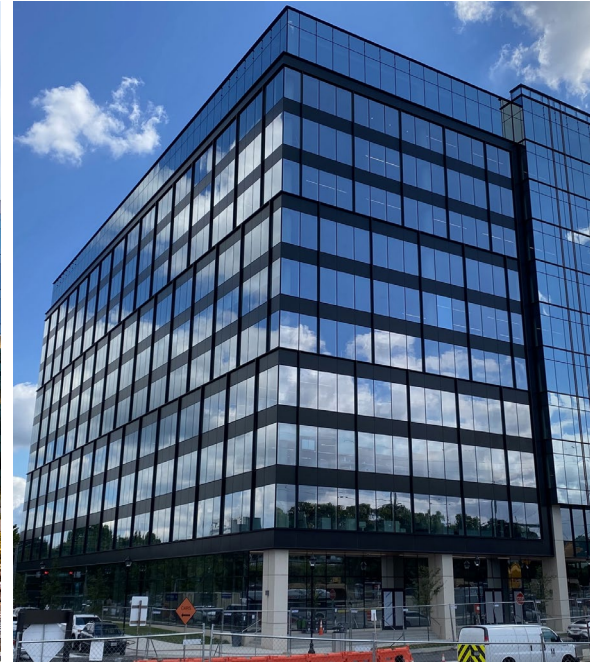
Metro Office at New Carrollton 329,000 SF Urban Atlantic/Bolton Development
