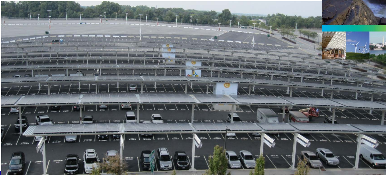
2 MW system at FedEx Field, September 2011
