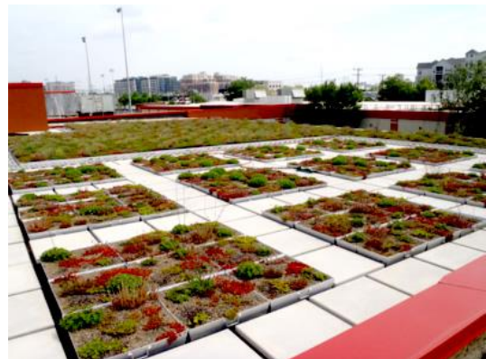
(Above: Green roof in Alexandria, VA)
