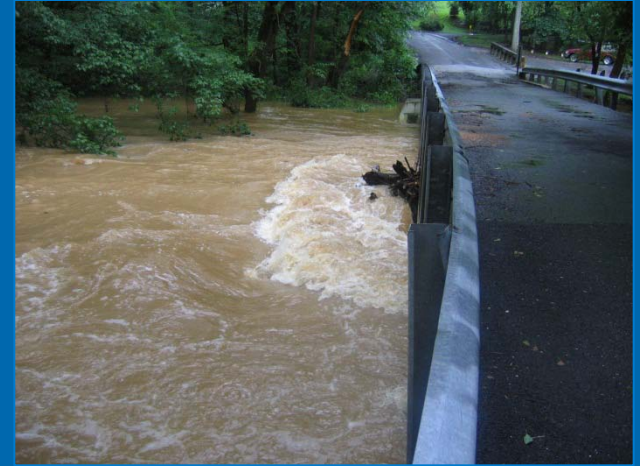
Floating Debris Lodged in a Bridge during Flood Event at Seneca Creek in Germantown, MD Photo Source: (FEMA/Skolnik 2006)
