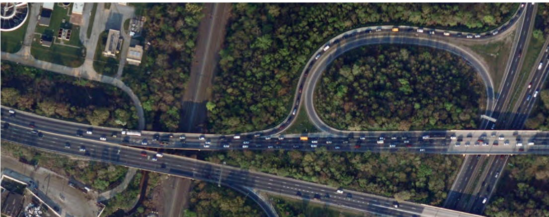
Photo Set Two: These photographs show the 2005 (top) and 2011 (bottom) configuration of the DC 295 bridge across the Northeast Corridor railroad right-of-way; note the absence of a significant merge lane in the 2005 photograph, and the friction that caused for southbound traffic on DC 295.
