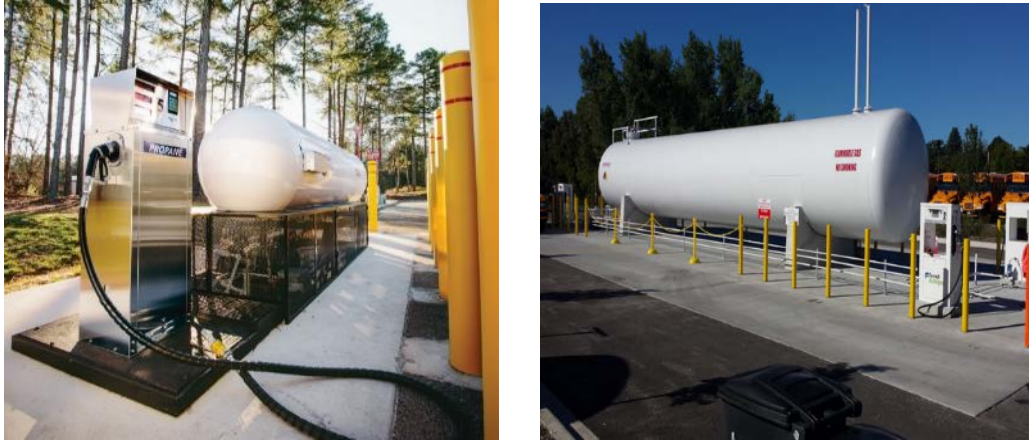
Figure 58. Propane autogas fuel stations are scalable from small, skid-mounted packages that include 1000-gallon tank, associated pumps, and dispenser with integrated fuel management system (left), to large built-to-order locations with 18,000-50,000 gallon tanks, multiple dispensers and separate fuel management/payment processing unit (right). Propane autogas fueling stations are governed by NFPA 30A standards governing all fuel stations.
