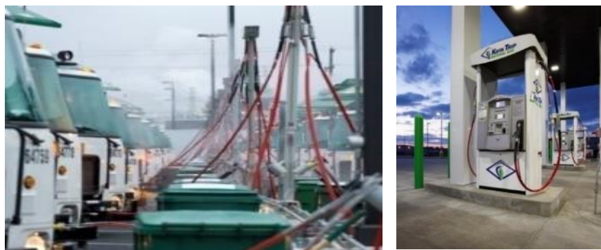
Figure 45: Time-fill Versus Fast-fill Refuse fleets are well-suited to time-fill fueling (left) because they typically sit idle overnight. CNG fast-fill dispensers for public access (right) are required to be National Conference of Weights & Measures-certified.
