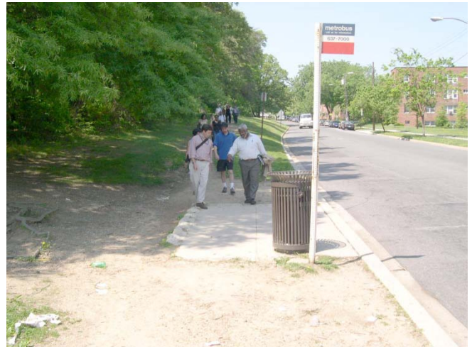
Figure 1: Missing sidewalk near Ft. Totten Metro
