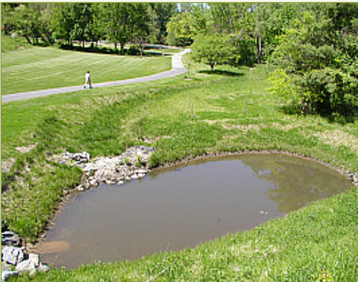
Stormwater Retention Pond
