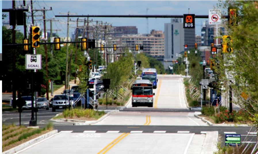
Median Bus Lane – Alexandria, VA
