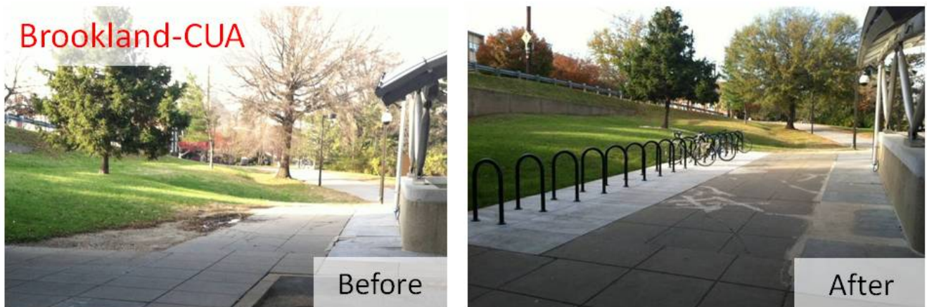
Figure 11: New Bike Racks (WMATA photo)
