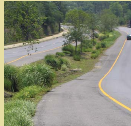
Low impact development median absorbs stormwater runoff from Adelphi Road in Prince George's County, Maryland.
