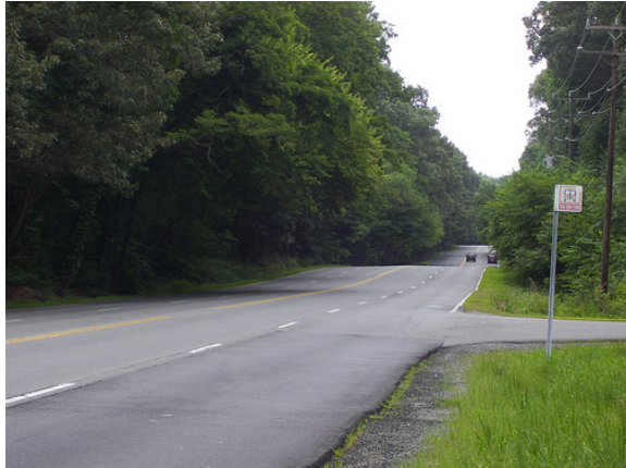
Figure 71: Lawyers Road Before Road Diet/VDOT
