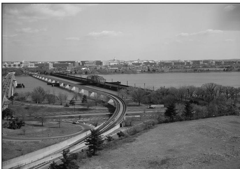
The Long Bridge, built in 1904, crosses the Potomac River and serves as the only freight connection between the District and Virginia. Photo courtesy of the Library of Congress Prints and Photographs Division Washington, DC.
