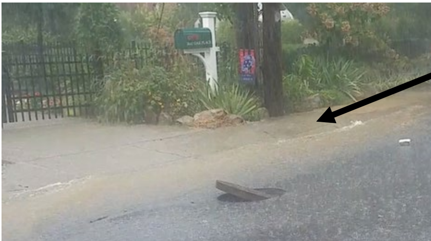
High-intensity events exceeding storm drain inlet capacity result in localized flooding impacts
