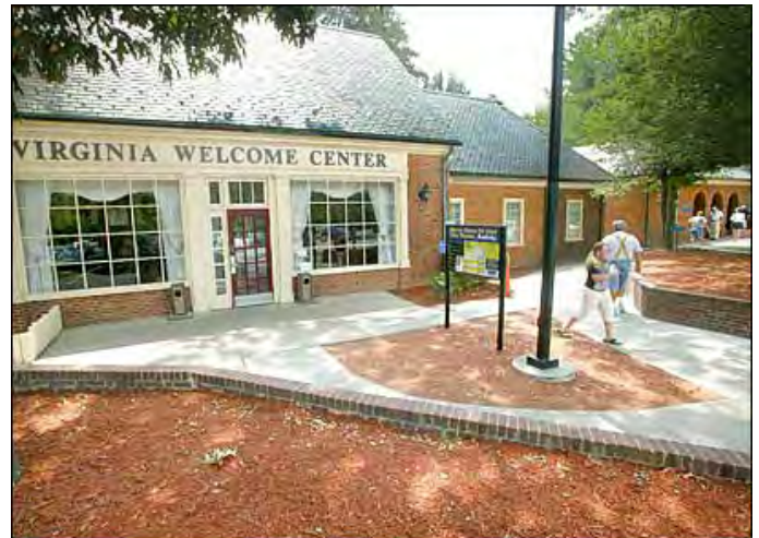
Skippers Safety Rest Area/Welcome Center - I-95 North at Mile Marker 1 (Source: VDOT Travel Center)
