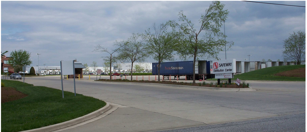
Figure 2.29 Safeway Distribution Center, Upper Marlboro, Maryland
