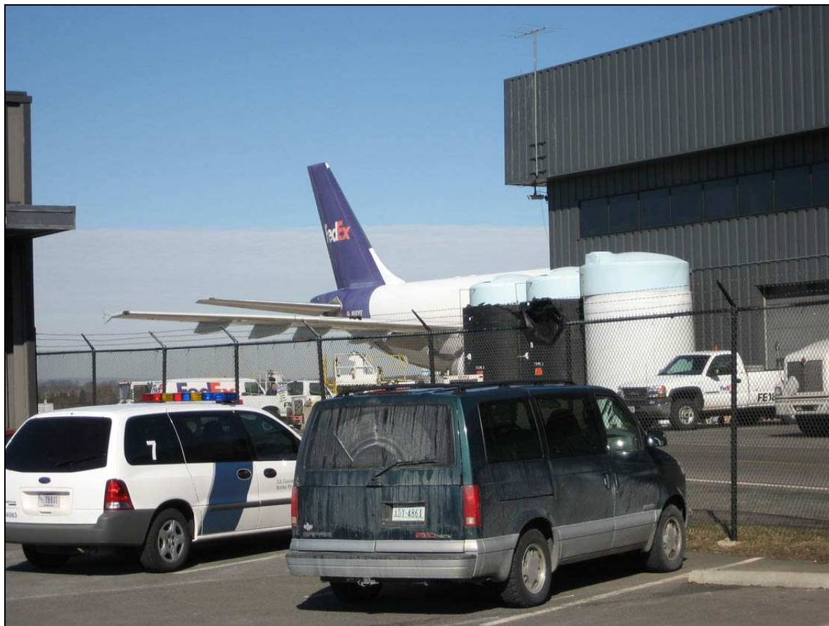
Figure 2.19 Dulles Airport FedEx Facility
