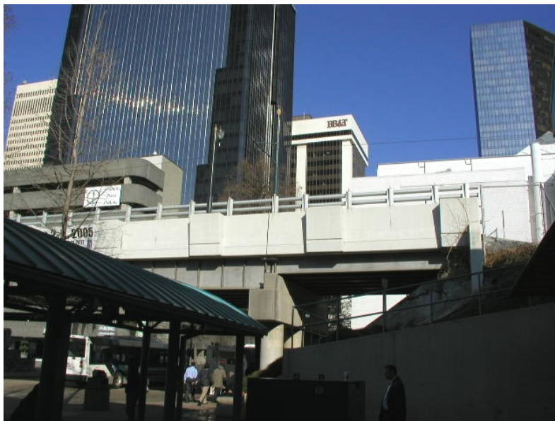
4th Street Overpass at Transportation Center
