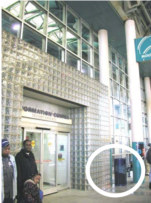
Location of Blast Can
