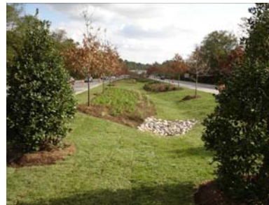
Bioretention in median: Prince George's Co.
