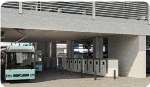
3. (10) 180 kW, (1) 360 kW BEB Chargers (5) 15 kW EV Chargers
