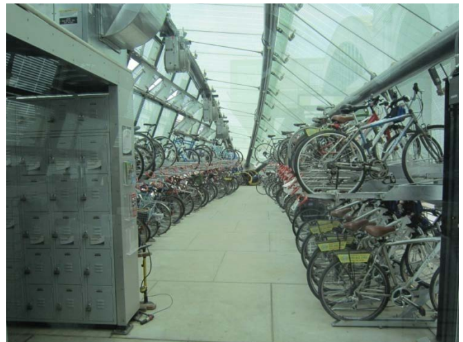
Figure 9: DC Bike Station Interior
