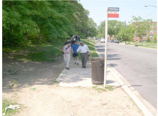
Figure 1: Missing sidewalk near Ft. Totten Metro
