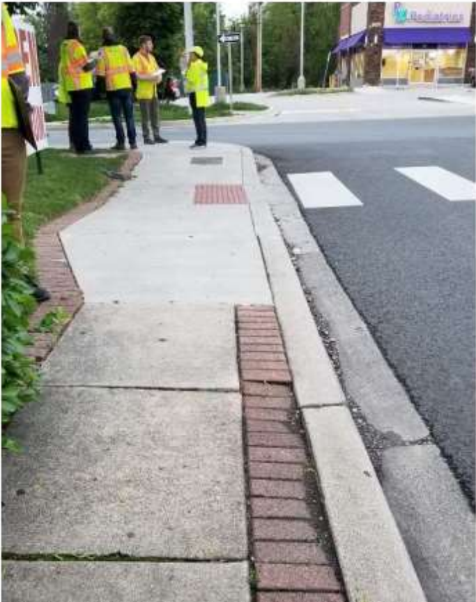
Deteriorating sidewalk
