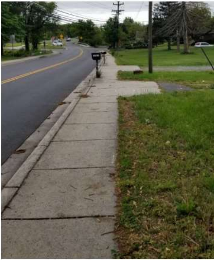
Sidewalk pinch point (mailbox)
