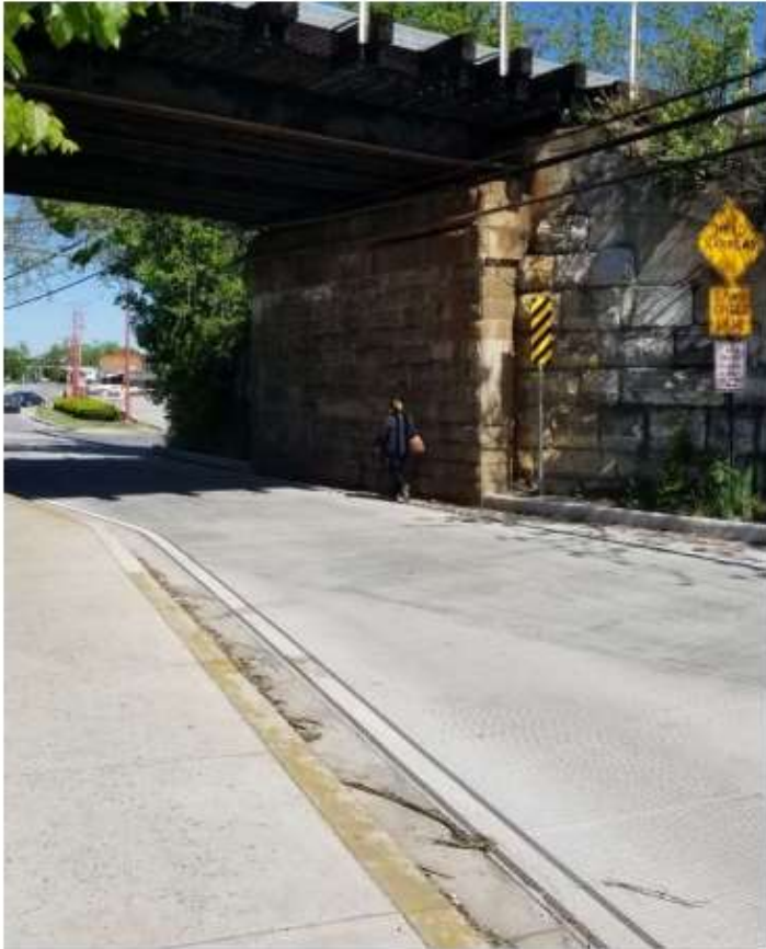
Pedestrian not using sidewalk under CSX railroad bridge
