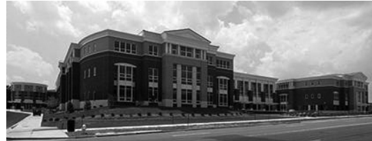
TC Williams High School in Alexandria adheres to LEED standards, and was recently awarded a Green Innovation Award for Best Institutional Project from the Virginia Sustainable Building Network. Its environmentally friendly features include a rooftop garden to provide stormwater management, waterless urinals, a 450,000-gallon underground cistern to collect and store rainwater for use in toilet flushing, and a system for tracking water and energy use.
