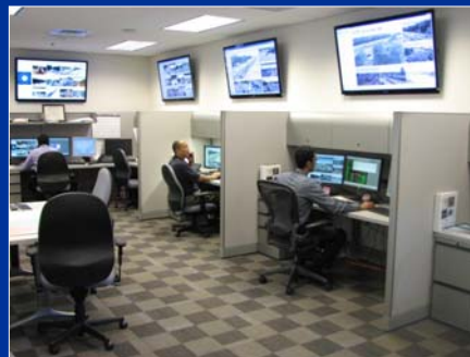
Signal Operations Center (SOC)
