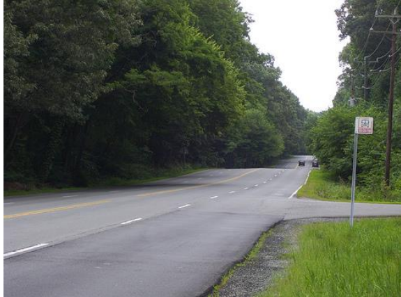
Figure 58: Lawyers Road Before Road Diet/VDOT
