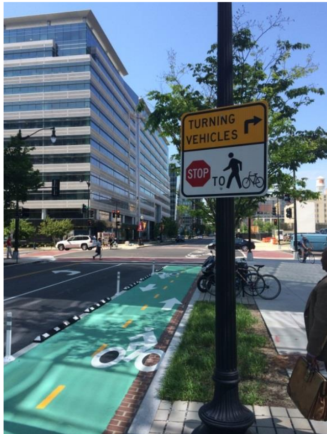
Figure 25: 1st Street NE Protected Lane/TPB/Michael Farrell
