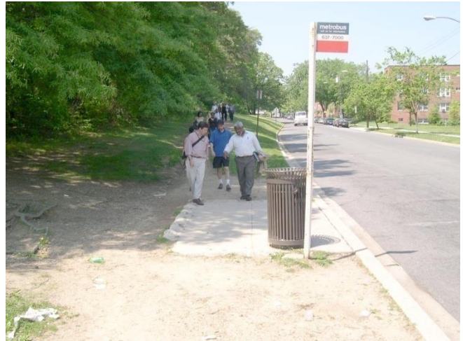
Figure 47: Missing Sidewalk/TPB/Michael Farrell
