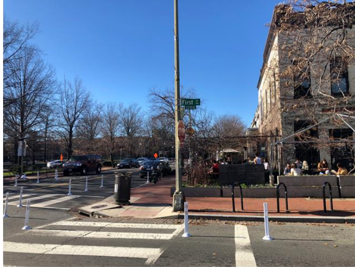
Figure 32: Flexpost Bulbouts/TPB/Michael Farrell
