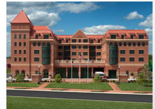
Fire Station at Potomac Yards – Earthcraft certified + LEED CI Silver (awaiting certification, 2013)
