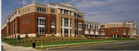
TC Williams H.S. – LEED NC Gold, 2009
