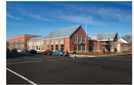
Charles Houston Recreation Center – LEED NC Gold, 2010
