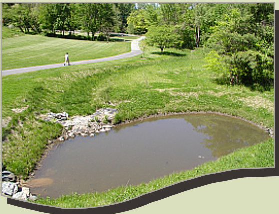
Stormwater Retention Pond
