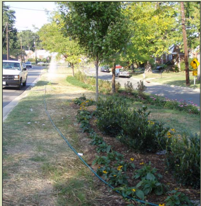
Local government stormwater programs are increasingly focused on infiltration of stormwater in public right of ways.
