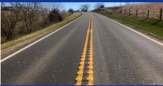
Centerline Rumble Stripe
