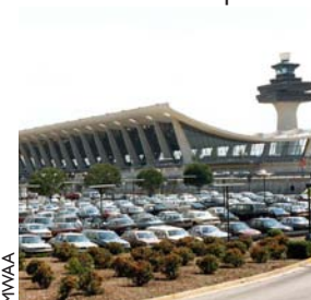
Dulles Corridor Rapid Transit
