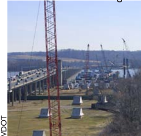
Woodrow Wilson Bridge
