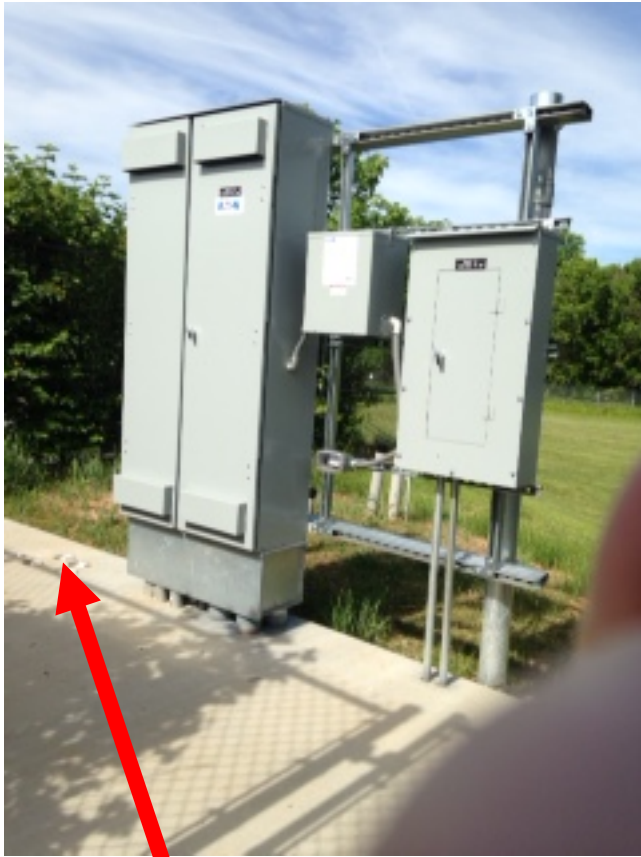
Conduit for future 10 stations & generator capped off
