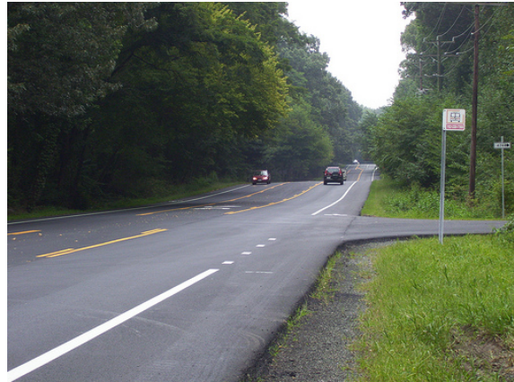
Figure 72: Lawyers Road After Road Diet/VDOT
