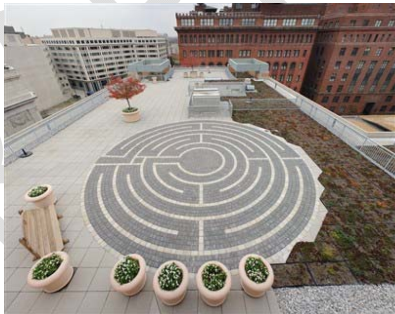
WRI green roof (Source: www.apabuilding.com )
