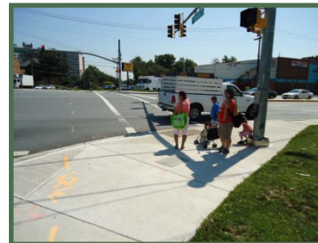
MDSHA Piney Branch Rd & University Blvd Intersection Improvements (2009)
