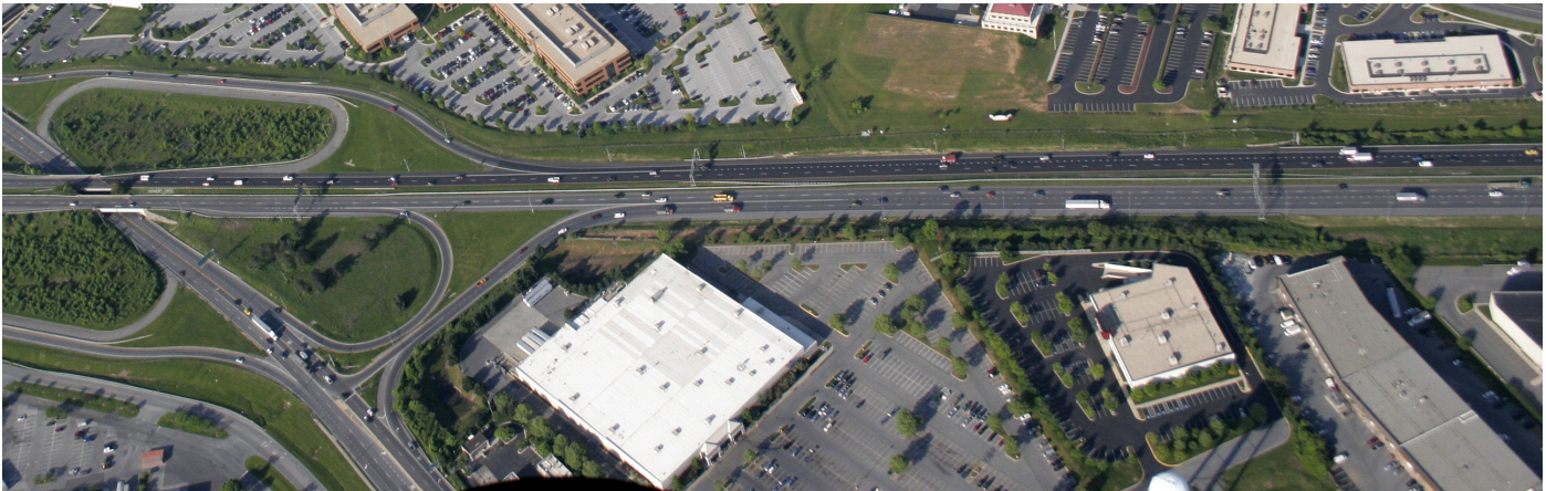
This photo shows typical 2008 peak-hour traffic conditions along the extended auxiliary lane between I-70 (off the photo to the right) and the MD 85 interchange (Buckeystown Pike, shown). This relatively minor improvement eliminated a major bottleneck from eastbound I-70 to southbound I-270.
