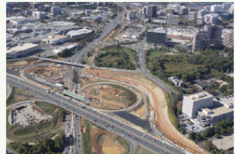
HOT Lanes and Dulles Rail construction
