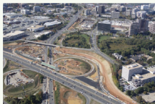
HOT Lanes and Dulles Rail construction
