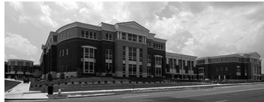
TC Williams High School in Alexandria, VA adheres to LEED standards, and was recently awarded a Green Innovation Award for Best Institutional Project from the Virginia Sustainable Building Network. Its environmentally friendly features include a rooftop garden to provide stormwater management, waterless urinals, a 450,000-gallon underground cistern to collect and store rainwater for use in toilet flushing, and a system for tracking water and energy use. The City expects to save $30,000 annually in potable water costs as a result of these measures.
