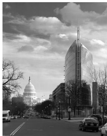
The National Association of Realtors' new Washington headquarters building has been awarded a LEED Silver certification for a high level of environmental performance. The striking, glass-wrapped structure was the first newly constructed building in the District of Co-
