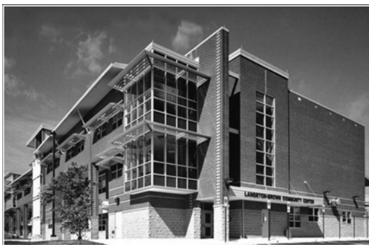
The Langston-Brown School and Community Center in Arlington, VA uses extensive interior daylighting with sunshades to control heating from the hot summer sun. Two large cisterns capture rainwater from the roof, which can be used for irrigation around the building. During construction, over 80% of construction debris was recycled.
