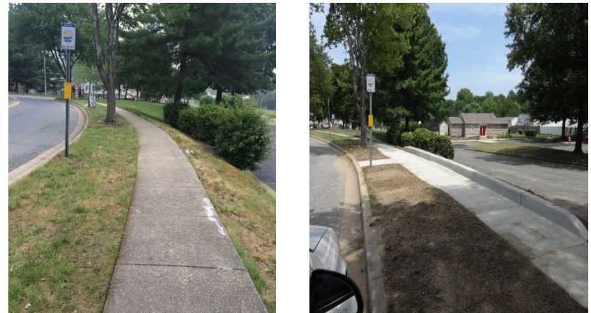
Nalley Road @ Nalley Court
